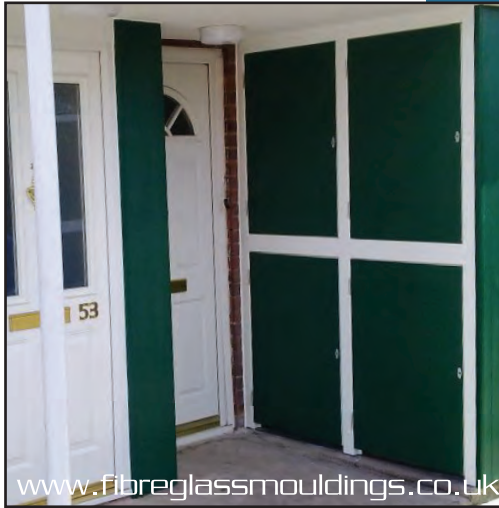
Bin Store Over Clad
